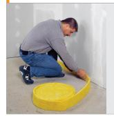
Place the perimeter strip along the walls to avoid flanking acoustic transmission and to allow for differential movement.
