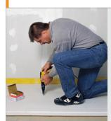
Secure the boards with Fermacell Flooring screws at 200mm centres (18mm screws for flooring under 25mm thick).
