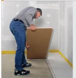
Lay the boards with the edges overlapping. Ensure there is a minimum overlap of 250mm at joints avoiding cross joints.
