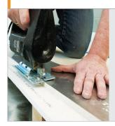
For the 1st row remove the overlap on the leading end and edge on the first and last sheet in the row, remove just the leading edge of the intermediate boards to ensure a tight fit against the perimeter strip.
