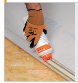
Apply Fermacell floor glue to the edges of the boards.
