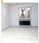
Allow 12 hours for the Floor Glue to dry and remove the excess with a scraper. Senso will take over from this stage and install their resin flooring onto the boards.
