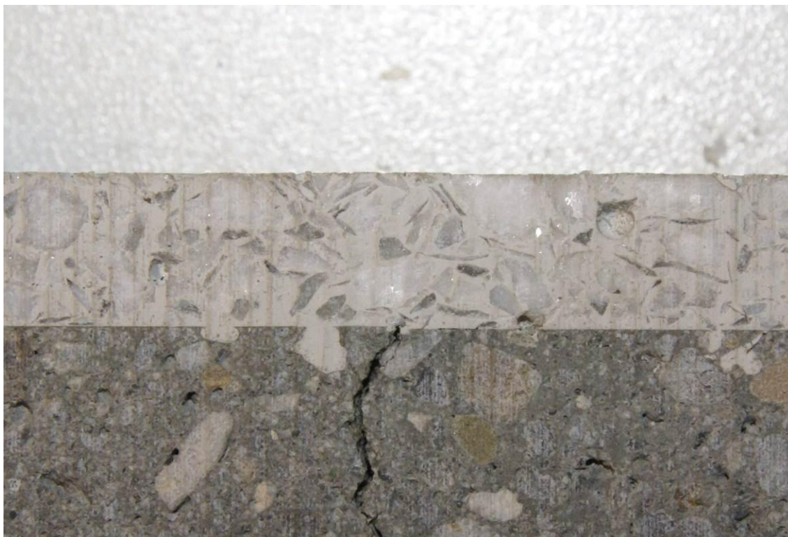
Photo 7, No crack development over a 0.4 mm wide crack after 6 hours in the additional test.
